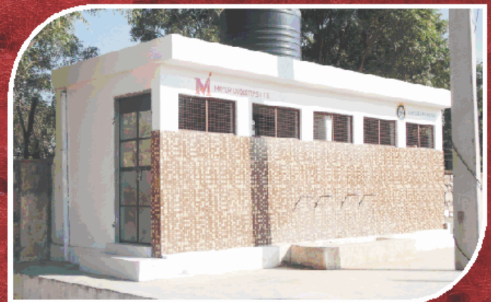
Constructed New Toilet (Apni Azadi)
