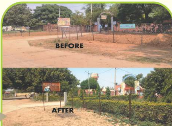
Renovation of Govt. School, Bhojlaw Garden
